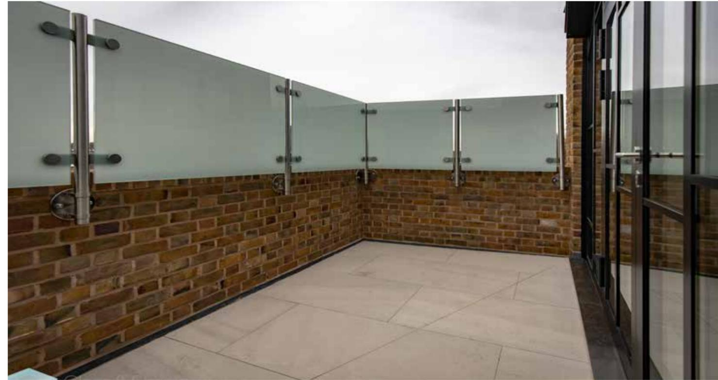
Installing a number of external glass balustrades for a private development in Cabul Road, London, provided a unique and original job for Glass & Stainless. Using 316 grade stainless steel throughout the glass clamps were attached to the 48dia x 2.6mm wall thickness posts to create a bespoke design for the project. Side fix brackets and posts were used to hold up 17.52mm toughened laminated glass that feature a 10% screen print for privacy.
